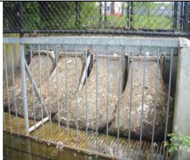
Figure 14: Capture of Organic Matter at the End of Storm Drain System
