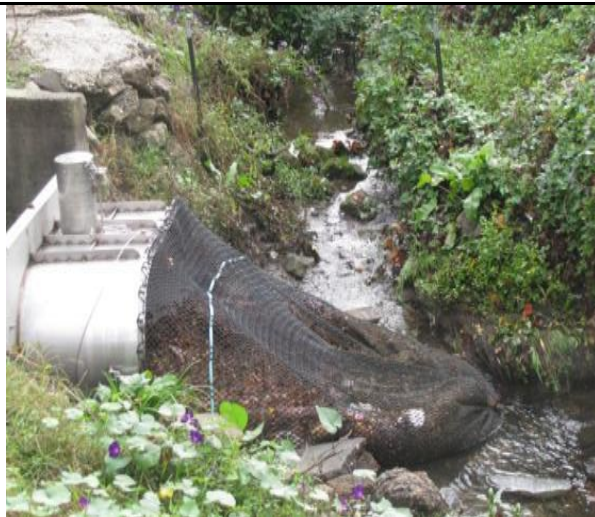
Figure 14: Capture of Organic Matter at the End of Storm Drain System
