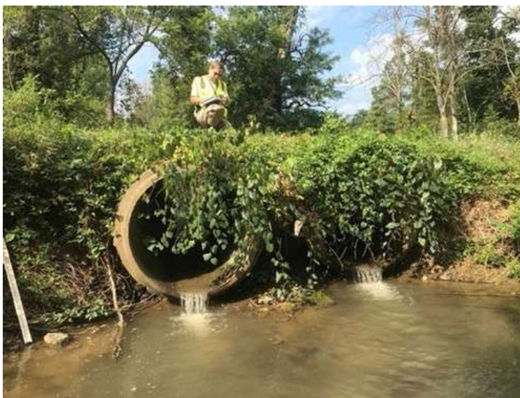
Figure 6. Outfall drop at Site 5
